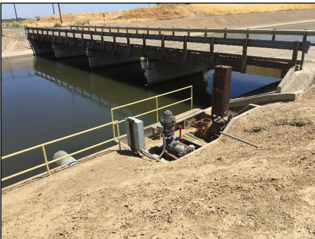
Lift / pressure pump at DM canal & Cottonwood Road
