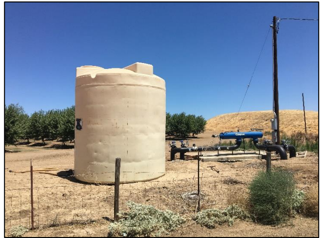
Filter station at SEC along Cottonwood Road
