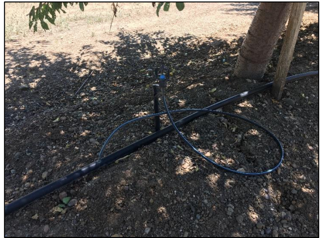
Irrigation water distribution line and micro-sprinkler
