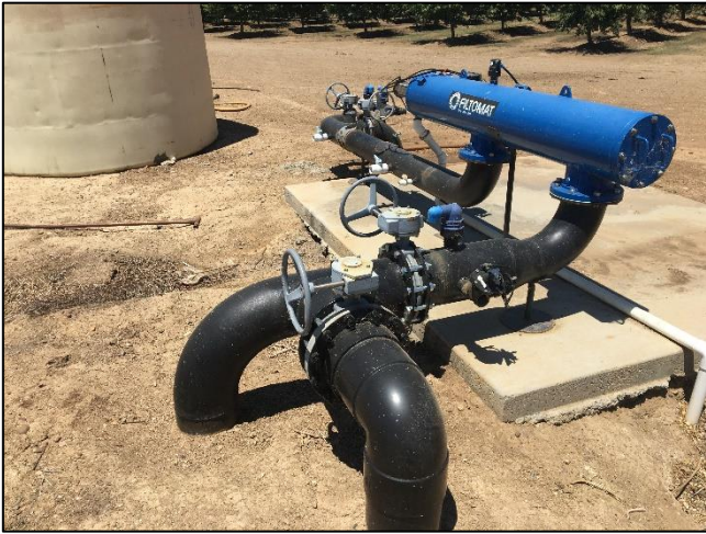
DPWD inlet and Amiad filter
